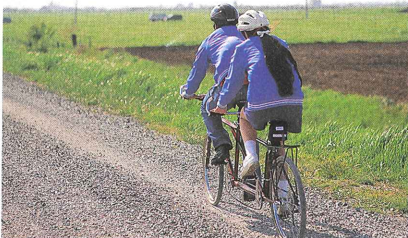
Figure 5-8 A Macadam road in Delta, BC. Macadam roads were later improved by the addition of tar to the surface layer of gravel. The resulting surface was called "tarmac."
